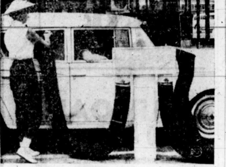
KEEPING COOL —Free air is supplied for car passengers, not tires, by an unusual cooling service offered by a drive-in restaurant at Fayetteville, N.C. Placed in an auto window by a carhop, a flexible hose pours in cool air drawn through underground ducts from a 30-horsepower air conditioning unit. A control in the hose outlet permits motorist to adjust the amount of cold air piped into the car.
