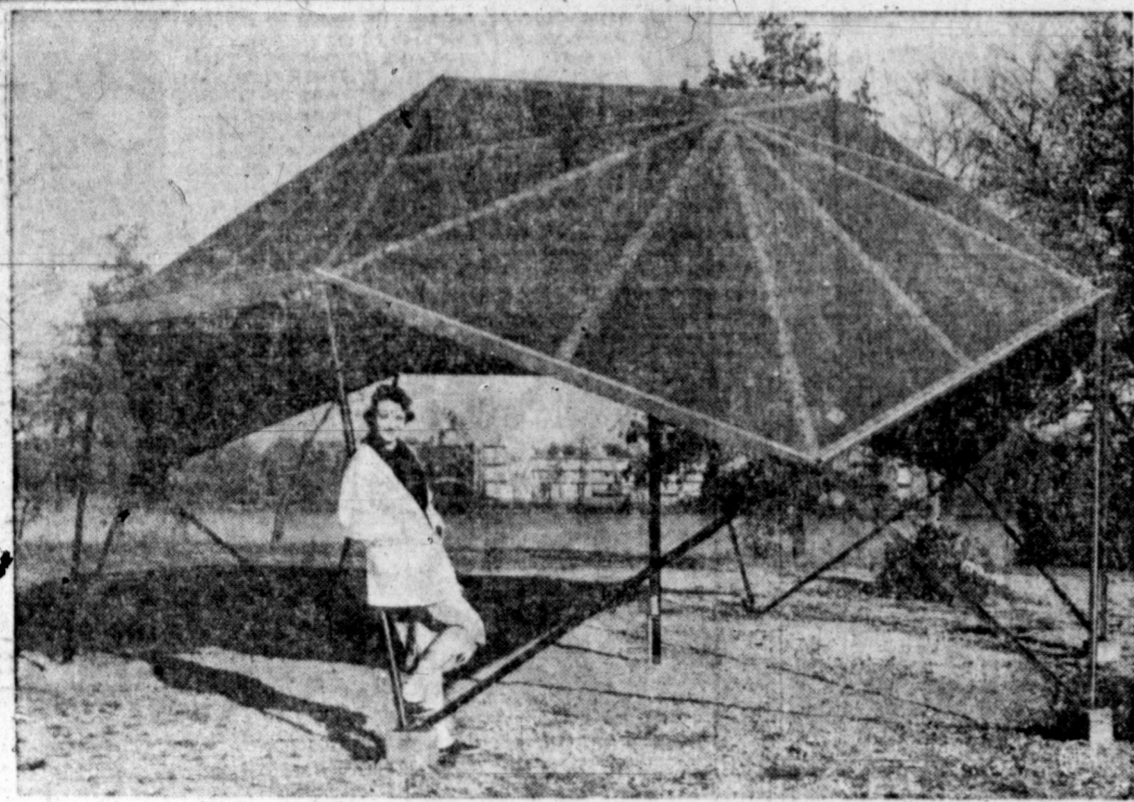
BUT NO WHEELS —Southern Illinois University at Carbondale has installed five of these plywood and steel geodesic domes on its grounds. They were designed by dome-inventor R. Buckminster Fuller, a research professor at the school. School authorities say the domes, to be used as picnic shelters, are supposed to take the undergraduate mind off automobiles which are being "phased out" of their campus lives.
