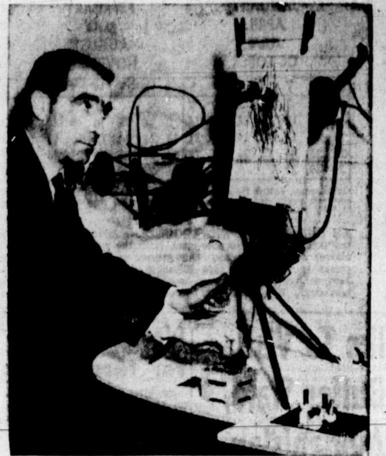
DOES IT MAKE CHANGE?—Inventor Jean Tinguely demonstrates his coin-operated painting machine in London. The user operates electric switches and mechanical arms holding tubes of paint and crayons mark up the paper on the easel. Result: a completely unpredictable abstraction.
