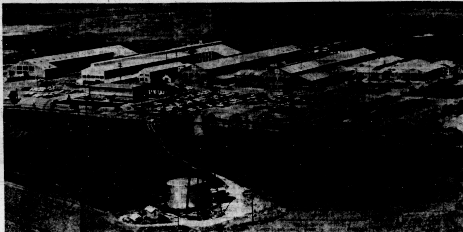
CABOT SHOPS OF PAMPA — The nation's largest producer of oilfield servicing units and third largest producer of pumping units is Cabot Shops, located six miles south of Pampa off U.S. 60. The Cabot plant currently employs 450 area residents. In the past 10 months the plants in addition to manufacturing drilling rigs, pumping and servicing units, has been producing of gun tubes for army ordnance.
