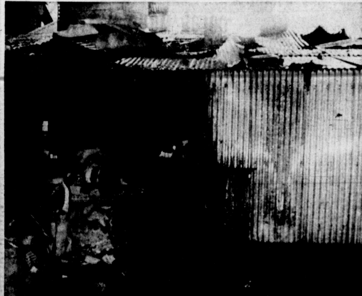
PAMPA FOUNDRY EXPLOSION — No persons were injured late Monday night when an explosion shattered the Pampa Foundry, 701 S. Somerville. Force of the blast, which occurred at 10:08 p.m., tore a sheet metal roof off the building's east side. Assistant Superintendent Roy Barnett said the explosion occurred when molten iron and slag poured from the bottom of a cupola furnace into a large puddle of water. James Conley, seen above near the still-warm cupola, said he and a number of fellow employees anticipated the blast and ran for cover. Barnett said the cupola should be ready for operations again this evening.
