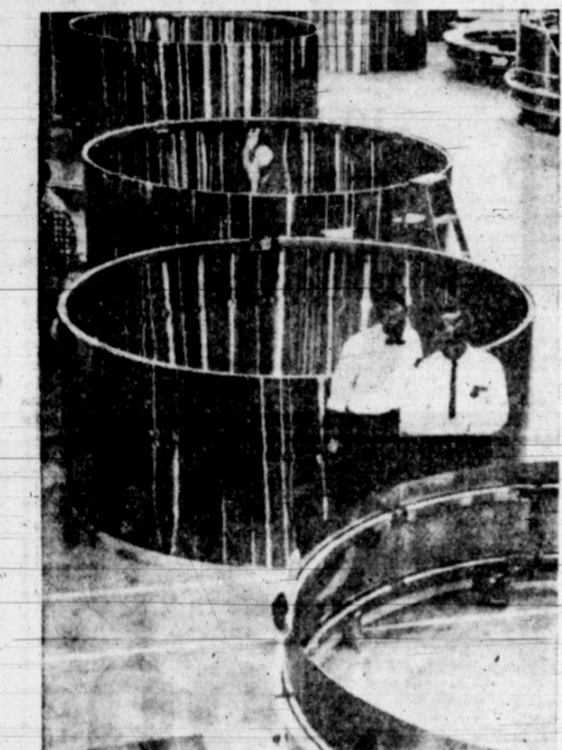
AT THE MISSILE WORKS—Engineers check work on gleaming bands of stainless steel in San Diego, Calif., factory where the Atlas ICBM is manufactured.
