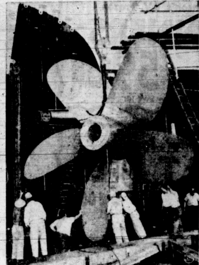
ATOMIC PROP —Using a crane, workmen ease the propeller of the NS Savannah into place in Camden, N.J. The Savannah will be the nation's first nuclear merchant ship. The ship is powered by a 2,500-ton reactor system.
