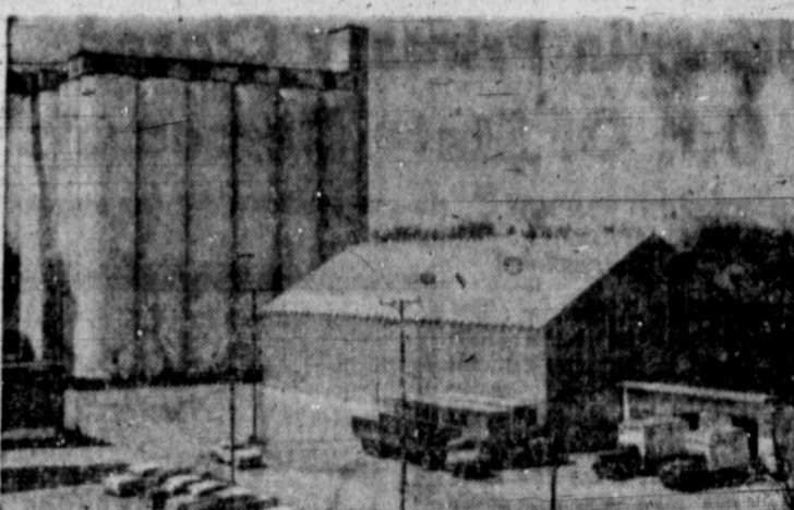
MAKING ROOM FOR MORE—This stark, angular structure is taking its place beside the stately concrete silos that have long been a landmark in the grain belt. It is a metal building recently constructed by the Missouri Farmers Association in Mexico, Mo. It was built to serve farmers storing grain under government loan and has room for 250,000 bushels. Storage of federal farm surpluses is now the number one business of private grain warehouses, under the watchful eye of the Commodity Credit Corporation. Cost to the government for storing grain during fiscal 1959 is estimated at 422 million dollars. It is expected to rise to 558 million in 1960.
