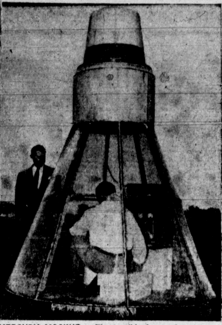
MERCURY MOCKUP — The possible home of a future spaceman, this object is a full-scale antenna-test mockup of a Project Mercury capsule. Engineers are shown testing the complete communications system for the capsule in Cedar Rapids, Iowa. Objectives of Project Mercury are to put a man into space, recover the capsule and its occupant and investigate the capabilities of man in this new environment.
