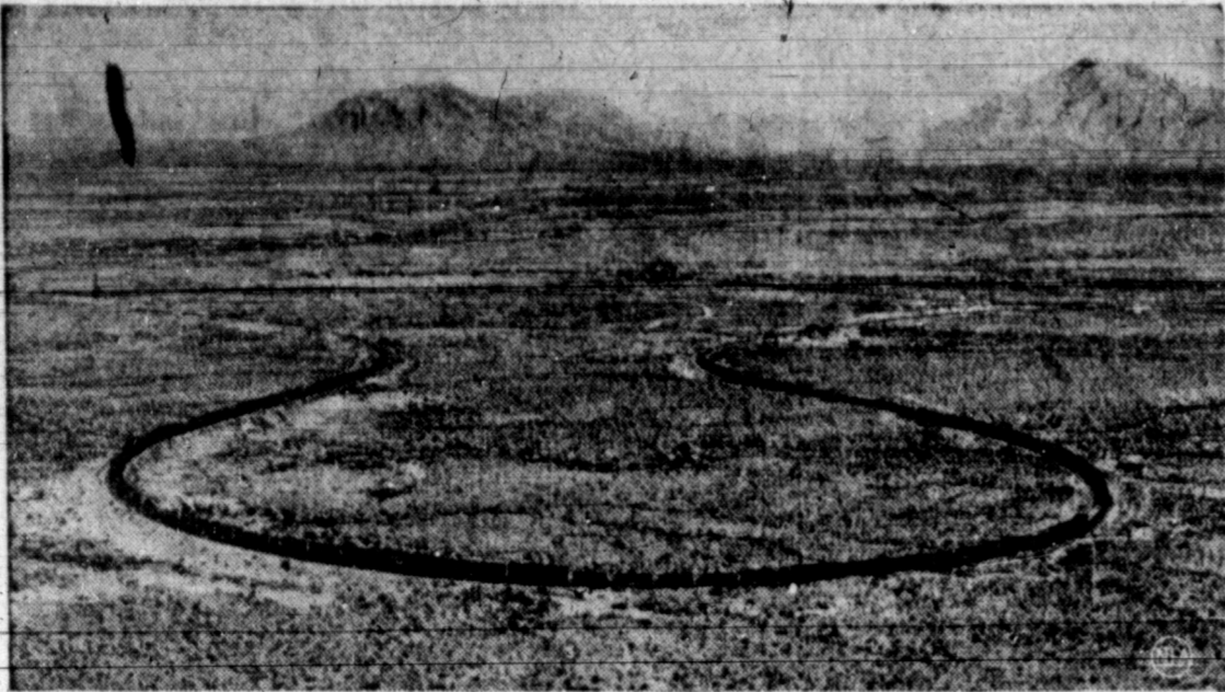
DESERT'S VANISHING IMPRINTS—Horseshoes are disappearing in the West these days. So with this famous horseshoe loop of the Southern Pacific 80 miles from El Paso, Tex. Slated for straightening, the meandering track was originally built that way to help freight trains up a 35-foot grade.
