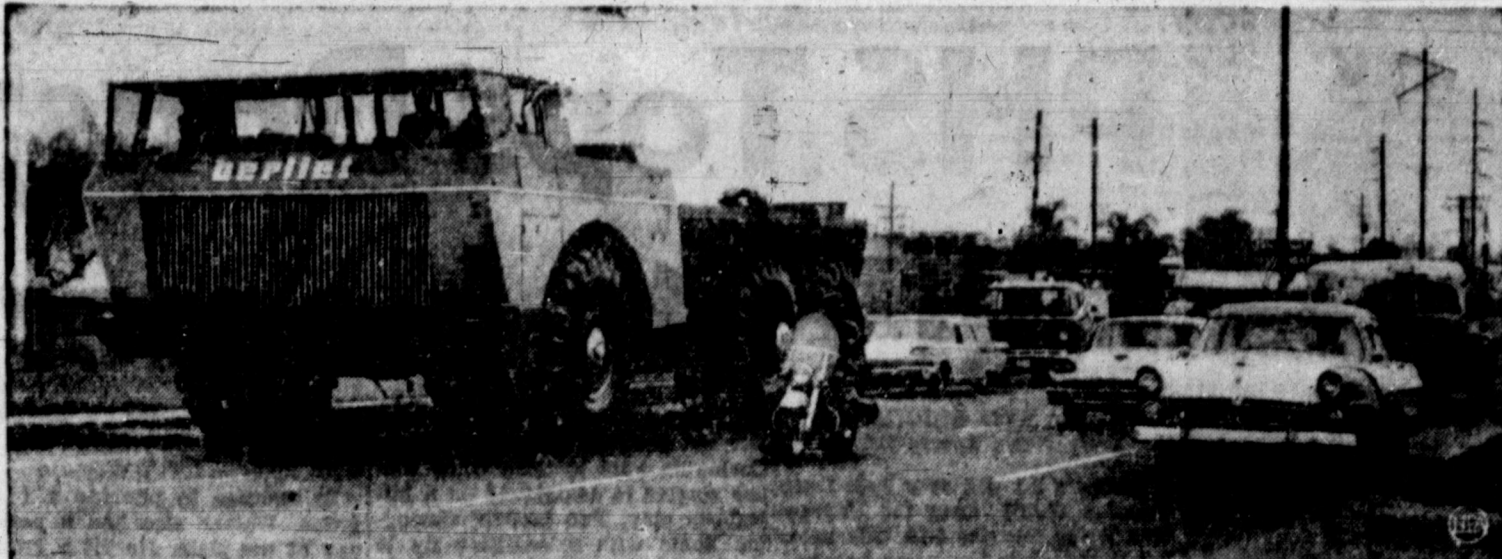
BIG CAMEL-FOOT TRUCK —The world's biggest commercial truck, dwarfing escorting police and autos in New Orleans, La. Designed primarily for off-the-road use, the truck is 16 feet wide, 13 feet high and 41 feet long. Specially designed low-pressure tires have ground pressure simulating that of a camel's feet, enabling the truck to carry 100 tons of material over all types of country. Made in France, it'll be displayed in Tulsa, Okla., May 14-23, at an international petroleum show.
