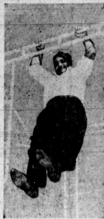
WEIGHT PULLING —Former world heavyweight boxing champion Rocky Marciano practiced chin-ups on his patented scaffolding at the headquarters of a new subdivision in West Palm Beach, Fla. The scaffolding is being used in the construction of a million-dollar homes exhibit.
