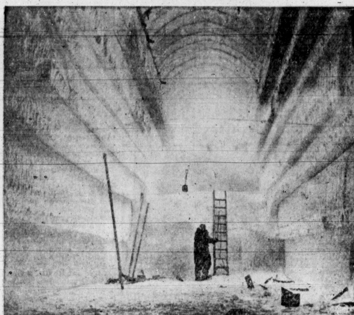
PALACE OF SNOW—A research worker seems tiny in a huge trench dug by the U.S. Army Corps of Engineers in the snow of the Arctic ice cap. The trench was roofed over by blowing processed snow over a temporary frame. When the snow hardened in a crust, the frame was removed. It is one of many trenches used as camps, workshops and storage spaces.
