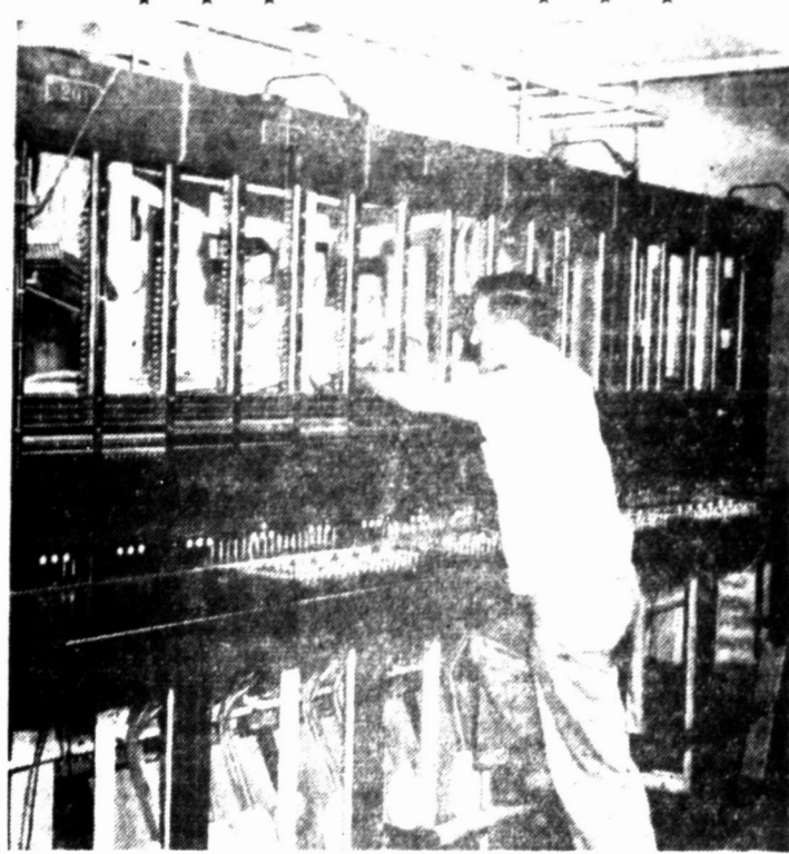
NEW SWITCHBOARD Units at the local telephone company, installation of which is now being completed, will boost the capacity from around 30,000 calls per day to 12,000 calls per day.
