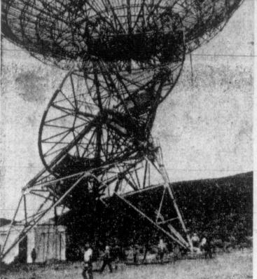
TUNING IN ON SPACE - A 200-ton, dish-shaped antenna takes shape in the Mojave Desert, Calif., as workmen continue work on a giant radio telescope at Goldstone Tracking Facility. The instrument will be capable of tracking space vehicles by radio signals as far as four billion miles from earth
