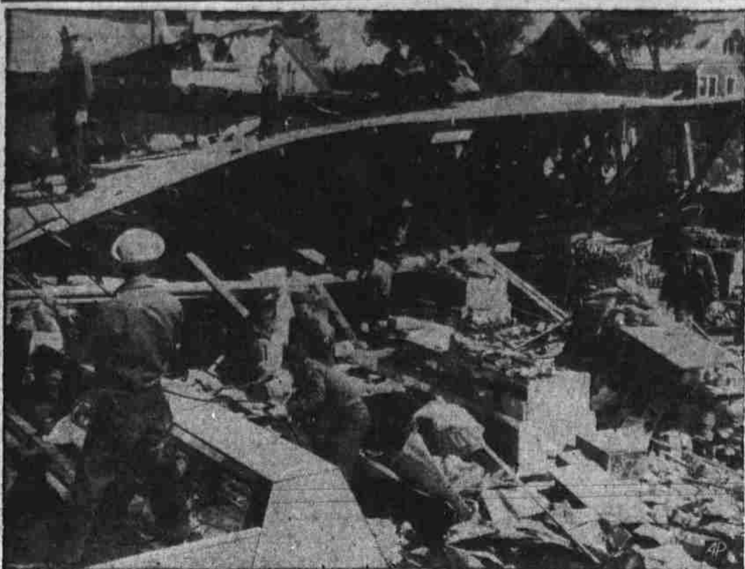
Store Collapses—A large, recently-built grocery store of the Safeway Stores, Inc., chain suddenly toppled into a mass of debris at Cheyenne, Wyo., Sept. 19, killing the mother of five children and injuring 11 other persons.
