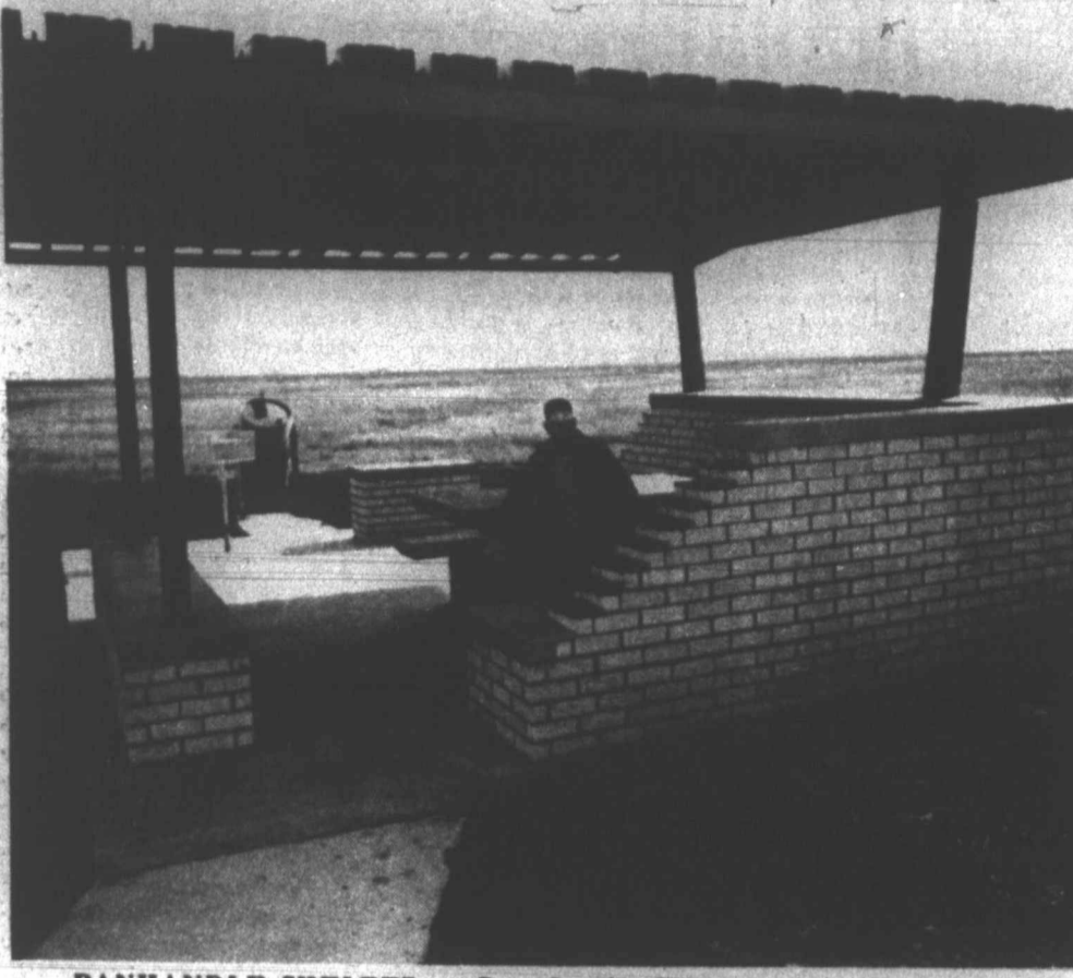
PANHANDLE SHELTER — Don Gandy, Texas Highway Department maintenance construction supervisor at Panhandle, rests inside one of the recently finished rest areas on U.S. 60. The arbor offers protection from the frequent Panhandle wind and a place to dine. (Texas Hwy. Dept. Photo)
