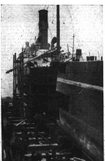
NOW, ABOUT MY OPERATION!—Gaping hole in the middle of this 250-foot tanker, "Comet," shown in drydock at River Rouge, Mich., marks the place where a new 74-foot section is to be spliced into middle, adding 12,400 barrels to her of capacity of 23,400. After girders and rivets had been removed powerful wineless yanked the ship apart.
