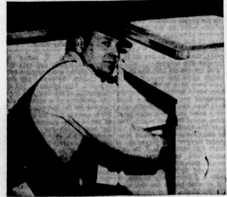
PLUMBING COMPLETED The final bit of plumbing work on the Optimist Boys Club building was completed yesterday and the opening of the newly-constructed building is nearing.
