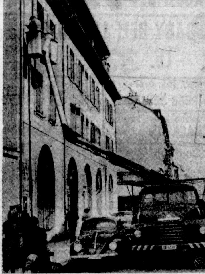
AUTOMATION ELEVATION —The long arm of automation is reaching out all over the world these days and Geneva, Switzerland, is no exception. A painter in the Swiss city, above, gives a drain pipe a new coat from the safety of a little box-like structure at the end of a hydraulic arm, controlled from the truck in the street below. Sure beats painting from a ladder.
