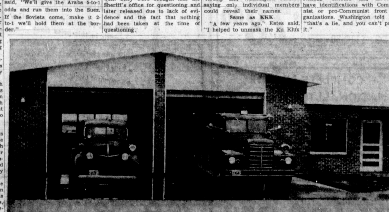
NEW FIRE STATION—Shown above is the exterior of the new fire station located at 17th and Aspen. The front of the new station faces 17th. At the present time two trucks are at the new station but when the other station, being built in the 1300 block of S. Barnes, is opened only the pumper at the right will remain at this station. Four firemen are on duty at all times at the new station. (News Photo)
