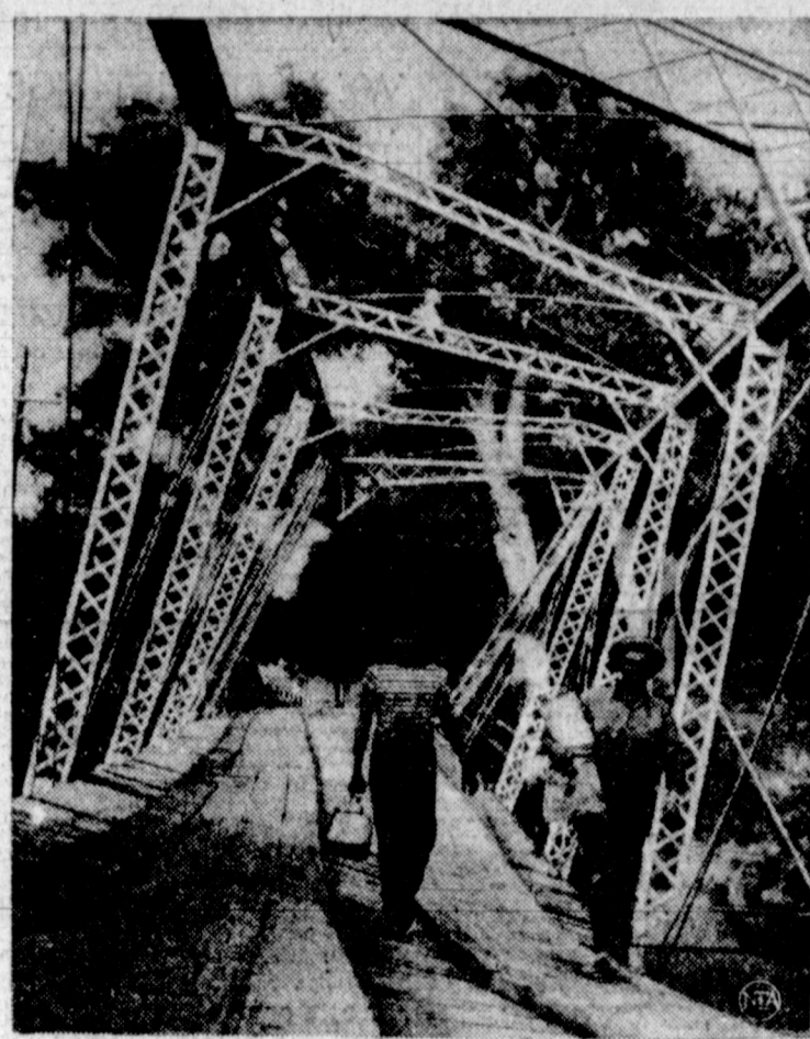
WON'T BURN THEIR BRIDGES —These two Minneapolis, Minn., men didn't burn their bridge behind them, but they might as well have, for the shape it's in. They have to park each day on one side of the Solomon River, walk across the bridge and take a truck to work. The bridge was hit by an auto and knocked askew. The men, Vince Pieschl Jr., left, and Don Charon take it all in stride.
