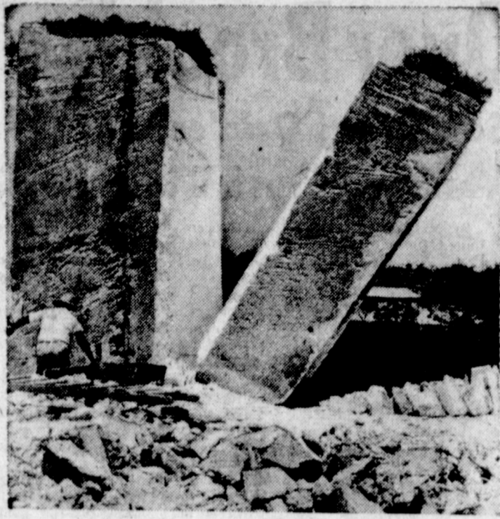
SAVED-OFF CLIFF —Sliced off neatly, this 25-foot piece of limestone coral topples to earth as worker at left stands clear in the 120-year-old quarry at Warwick, Bermuda. Though explosives, picks and shovels are normally associated with quarrying operations, the workers employed hand saws to cut the coral, used extensively in building on the island. This section, representing 27 hours of sawing, will be cut into smaller bricks.
