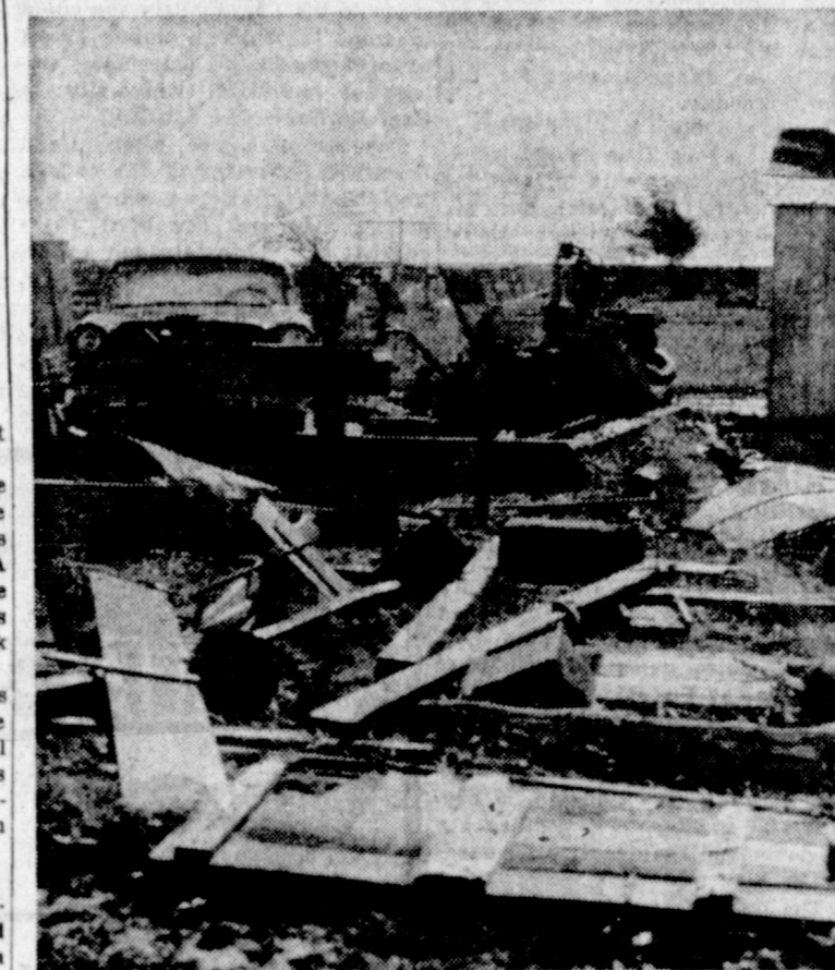
STORM DAMAGE—A portion of the damage at the John Sims place, located 10 miles northeast of Pampa on the Miami highway, that resulted from the tornado that struck there about 5 p.m. yesterday is shown. The car in the picture was inside of a shed that was blown away. All of the buildings were damaged and some of the metal and boards from the buildings was scattered for several hundred yards. (News photo)
