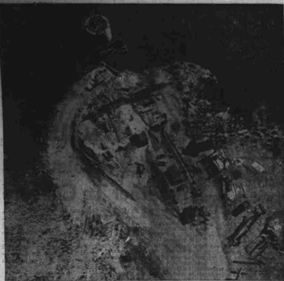
Getting Ready For Pump Station
