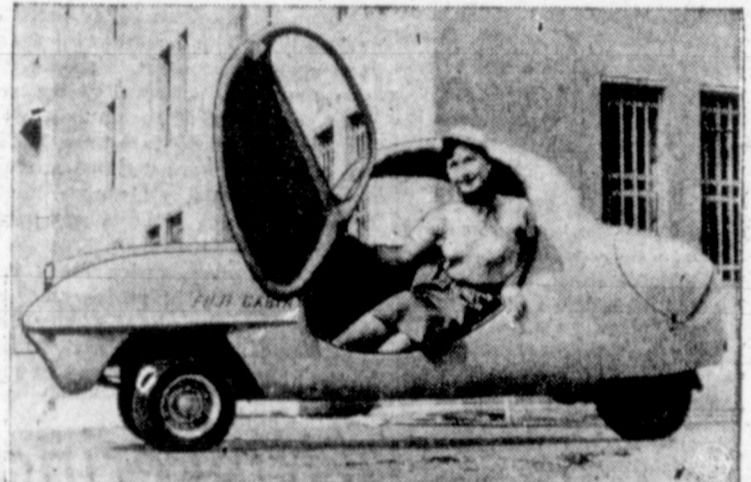
CABIN CLASS—Looks like a midget car, but it's a new three-wheeled plastic cabin scooter, recently displayed in Tokyo. The young lady demonstrating the door action is not standard equipment. Scooter has a 5.5 H.P., air-cooled single-piston engine which make a top speed of 37 M.P.H.
