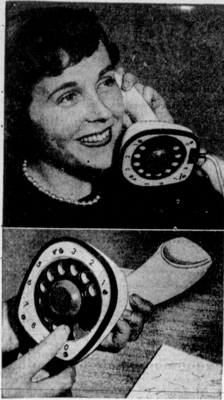
PHONE OF THE FUTURE?—A radically different one-piece dial telephone was recently demonstrated by its maker, the North Electric Company of Gallon, Ohio, to the Independent Telephone Association's convention in Chicago. At top, Claire Jensen shows how it is used. Bottom photo shows dial, built into the base. It is a one-piece receiver-transmitter which stands on its own 4 1/2-by-3 1/2-inch base which has a special "standswitch" button. When user lifts phone from table the button switches automatically to the "on" position.
