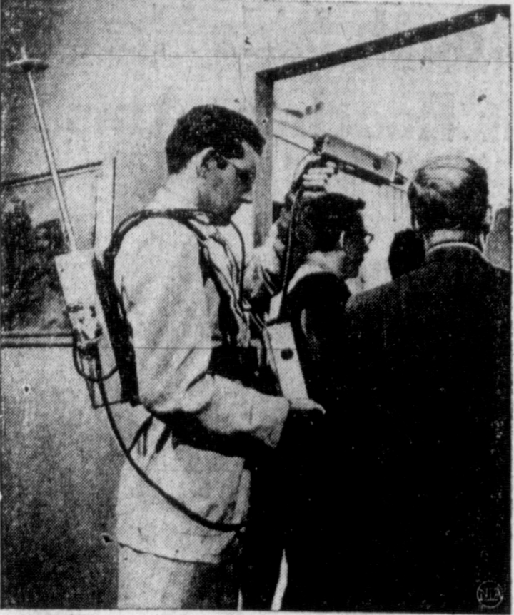
ONE-MAN TV —Unconventional equipment convention-bound is this lightweight television camera and transmitter. The portable gear, weighing only 19 pounds, will be used in covering the Democratic and Republican conventions. This new equipment, developed by RCA's David Sarnoff Research Center in Princeton, N.J., is said to be far more advanced than previous one-man models.
