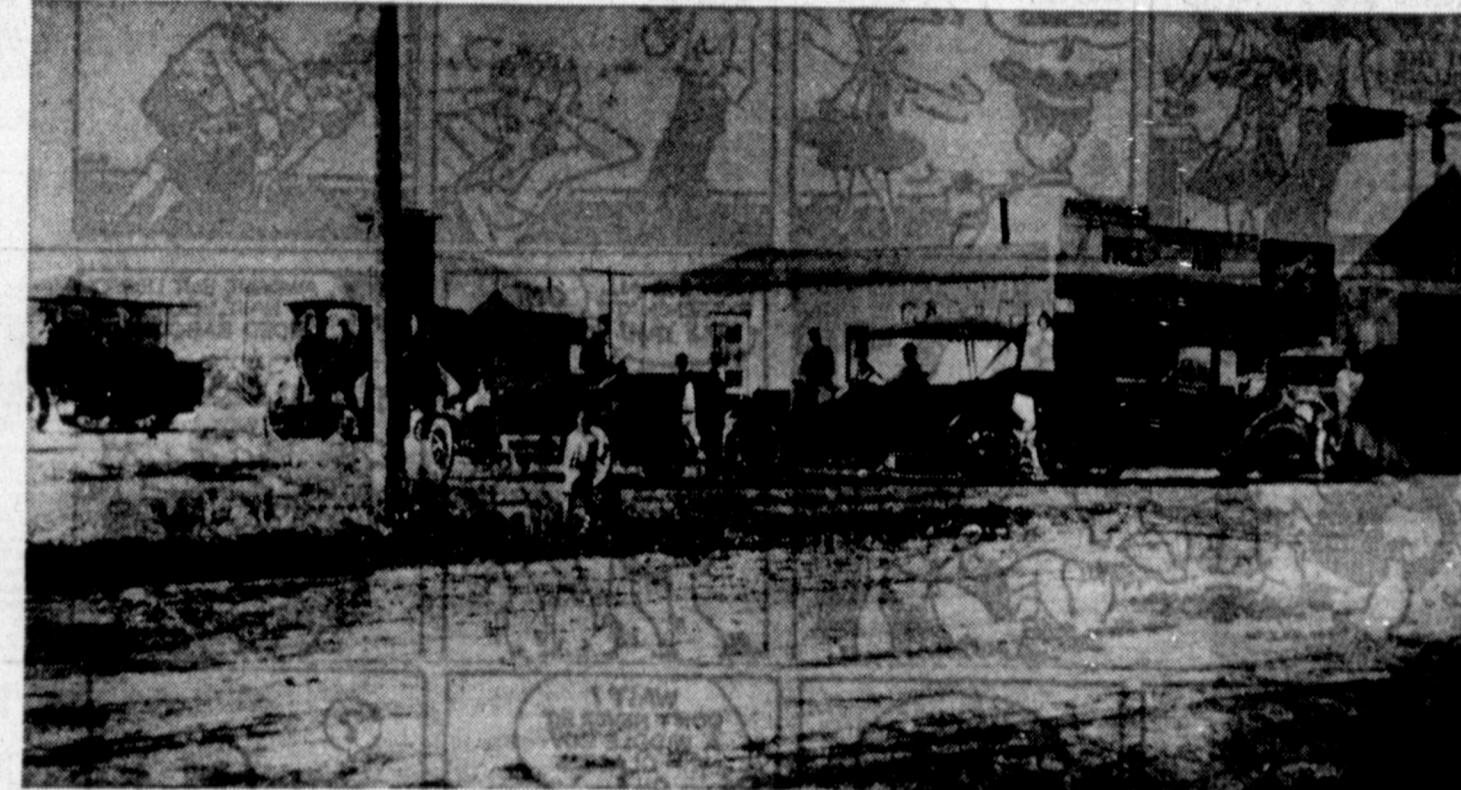
PAMPA GARAGE 38 YEARS AGO, 1918 — Then Pampa Garage was on the northwest corner of Foster and Frost, where the Hillson Hotel Building is now. In the background of the picture are the old First Baptist Church, and the red brick school house. Three persons in the picture have been identified as Les Saltzman, far right; Jud Wilson, second from right; and J. M. Saltzman, the boy in the central foreground facing the camera which was placed on the then unpaved Foster St. A copy of this picture is hanging in Pampa Garage & Salvage, 812 W. Kingsmill (4-5831). Lee Roy McBride, garage operator, invites every one to come in and help him identify those in the picture.
