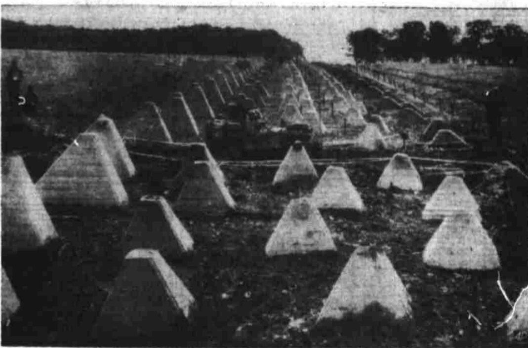
YANKS PENETRATE SIEGFRIED LINE BARRICADE—A machine-gun carrying jeep drives through a gap cut in reinforced concrete "dragon's teeth" barricade of the Siegfried Line inside Germany near Aachen as American forces advance into enemy territory. Peter J. Carroll, Associated Press photographer with the war still picture pool, made this photo. (AP Wirephoto).
