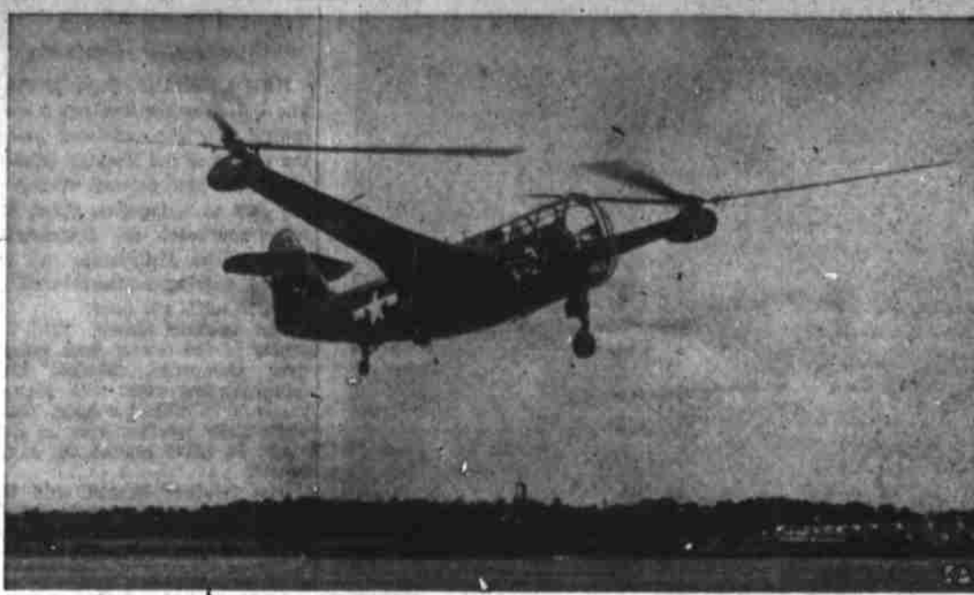
DUAL-ROTOR HELICOPTER—The Platt-LePage XR-1 helicopter, experimental Army model with two rotors, hovers above Wright Field, O., headquarters of the AAF materiel command.
