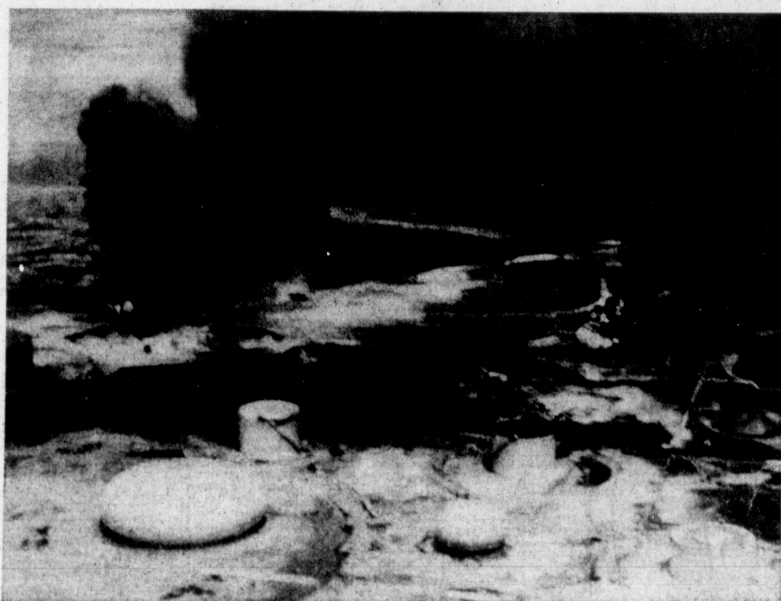
SMOKING INFERNO — Shown above is the storage tank area of the Shamrock refinery located near Dumas which was the scene of Sunday's explosion in which 19 were killed and 31 others were injured. The tank burning on the right of the picture is in the area where the explosion occurred and where most of the killed and injured were trapped. Three tanks were ruined by the explosion and one other had the contents burning but did not explode. (News photo by Fred M. Parker)
