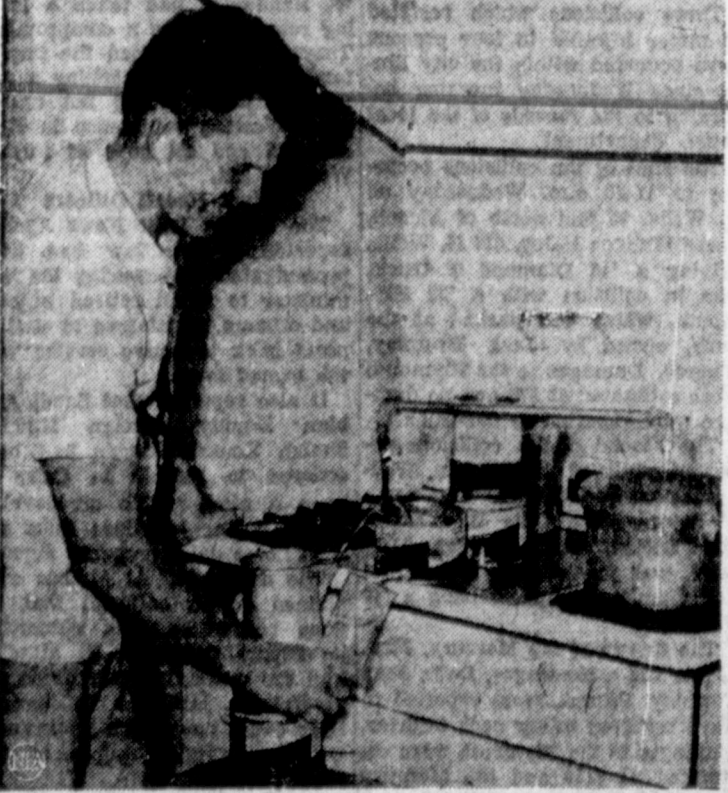
DOMESTIC DISTILLERY —Because of a drought in the local area, Dallas, Texas, has had to bring in water from the Red River. The complaint of residents is that the imported H 2 O is too salty. Davis B. Hilton, above, has solved that problem for himself. He's rigged up a pressure cooker, copper coil, a coffee can and an oil can to get salt-free water at the rate of one gallon per half-hour. Employing the process of distillation, Hilton converts salty tap water into the purest water in town.
