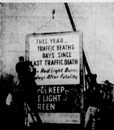
**"OPERATION LIFESAVER"**—Workmen erect a unique eight by 10-foot traffic warning and safety sign in front of the city hall at Orem, Utah, as part of the town's continuing safety campaign. Operated from a switchboard in city hall, the sign will show a green light as long as no accidents happen. When one does, the light changes to red and if there is a fatality, remains red for three days.
