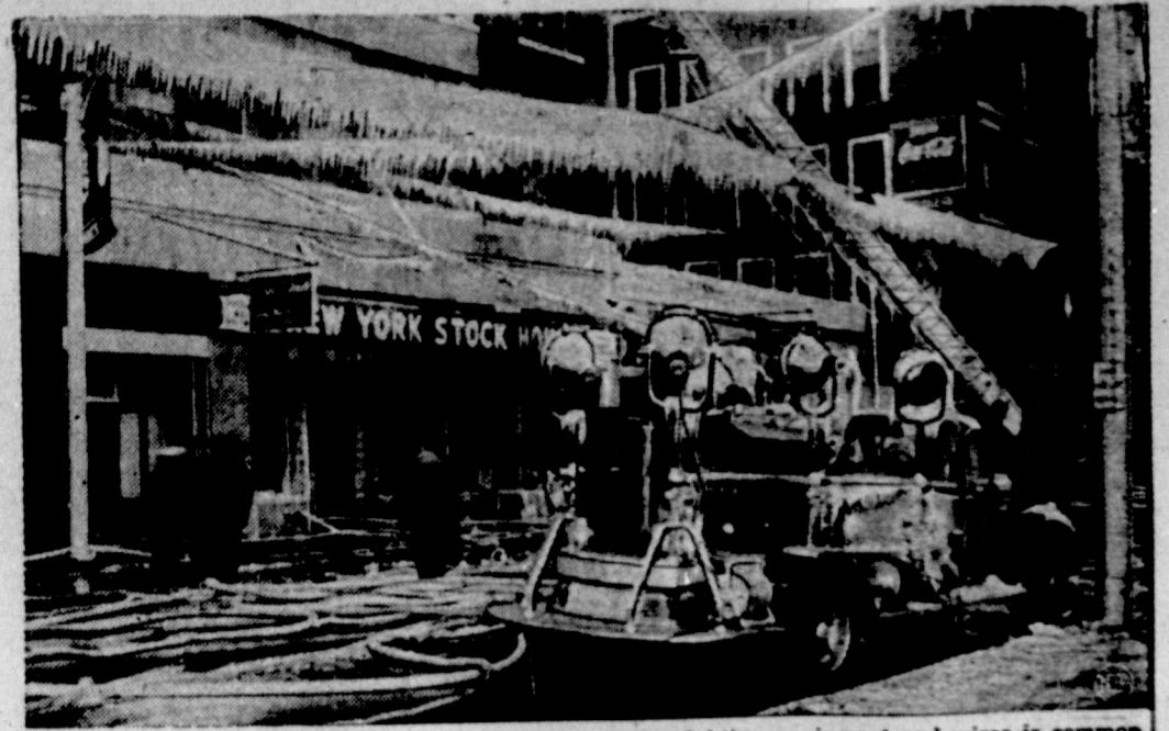
THE SUNNY WHERE? —The sight of ice-covered fire-fighting equipment and wires is common enough this time of year—except in the South. Proving that it gets cold there, too, is this picture taken in Atlanta, Ga. Temperatures were in the low 20's when firemen were called to extinguish the blaze at the New York Stock House, a clothing establishment.
