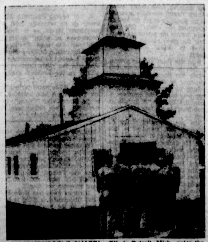
DO-IT-YOURSELF CHAPEL—G.I.'s in Detroit, Mich., enter the wooden chapel they built themselves. Members of the 18th Antiaircraft Artillery Battalion, they built it from donated materials.
