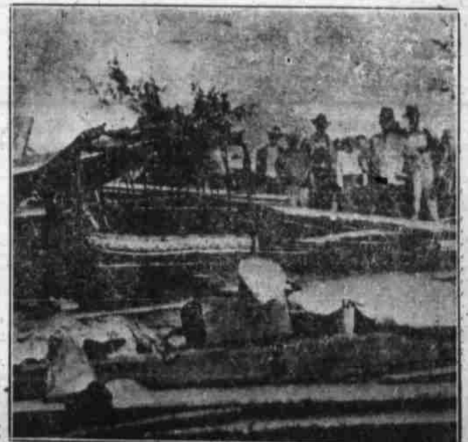
Two persons were killed in the wreckage pictured above when a storm of tornadoic proportions struck near Tulsa, Okla. The victims were Mr. and Mrs. Andrew Tackett. (Associated Press Photo.)
