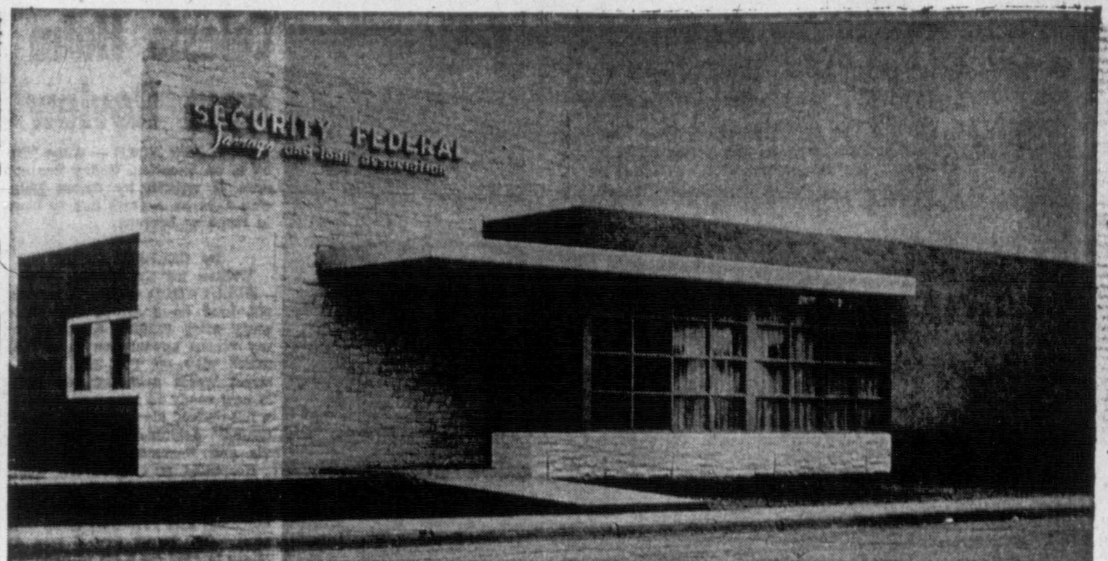
NEW LANDMARK — A new landmark for Pampa, Security Federal's new building is modern in style, inside and out. Construction features include brick and Austin limestone exterior, all year air conditioning, Terrazo and vinyl tile floors, luminous ceiling in work area, perforated Blonde Limba panel to reduce office machine noise, and many others.
