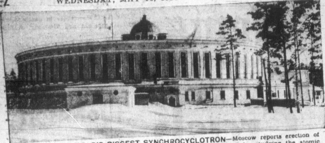
REDS BUILD WORLD'S BIGGEST SYNCHROCYCLOTRON —Moscow reports erection of the world's largest synchrocyclotron. The giant machine, designed for studying the atomic nucleus, was developed by the U.S.S.R. Academy of Sciences. The circular building, above, is the central block where the synchrocyclotron is installed. Its circular magnet weighs 36,000 tons and has a diameter of nearly 200 feet. Photo and caption material from Soviet sources.
