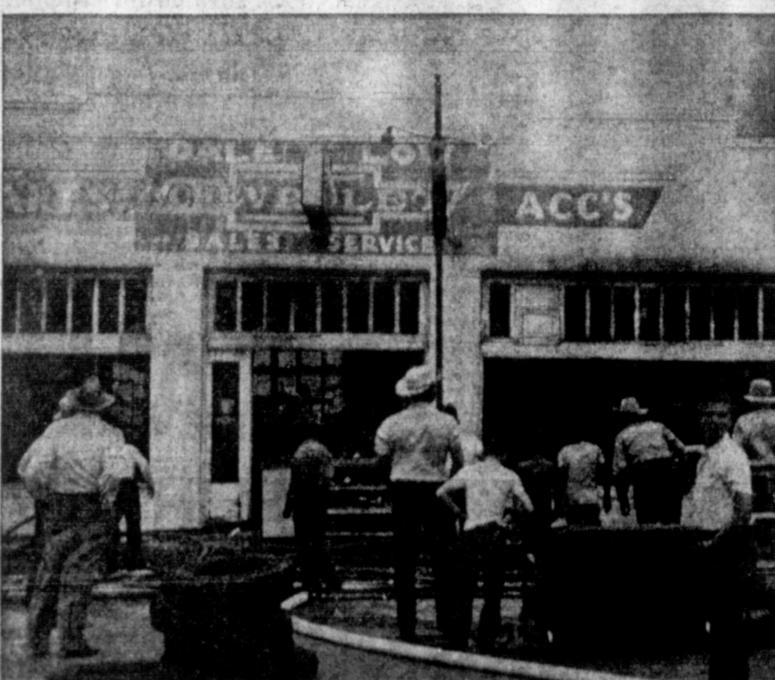
FIRE GUTTED BUILDING — Shown above is the Dale Low Chevrolet garage in Miami as firemen battled the fire that destroyed the firm Saturday night. The fire, of undetermined origin, was first noticed at 5:15 p. m. yesterday and was put out about 6:45 p. m. after the arrival of firemen from Pampa and Canadian. (News Photo)
