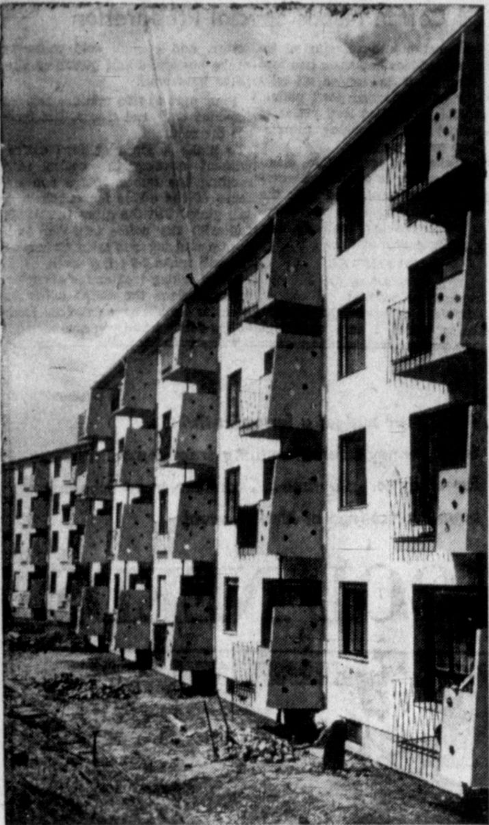
NO BALCONY SCENES HERE — The Berlin architect who designed this apartment house seems to have been hit by the Swiss influence — Swiss cheese, that is — in creating the balconies. Each balcony is well-protected from the sight of curious neighbors, while allowing light and air to get through.
