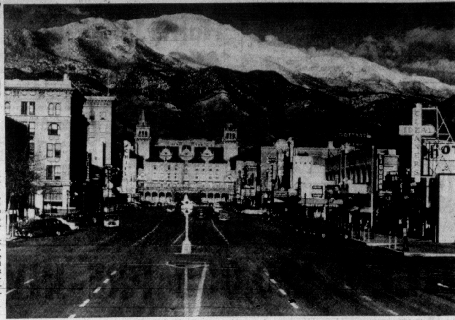
SNOW-CAPPED PIKES PEAK — Here's the famous peak viewed from Pike's Peak Avenue in downtown Colorado Springs. The mountain is only one of over 52 peaks in the state over 14,000 feet, and is perpetually covered with snow. In the foreground is the Antlers Hotel. (Photo by Stewart)
