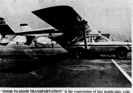
'DOOR-TO-DOOR TRANSPORTATION" is the expectation of this double-duty vehicle, the AVE Mizar. It integrates the airframe and pusher type engine of a Cessna Skymaster with a modified Ford Pinto. A two-minute operation connects or separates plane and auto. Testing is underway.
