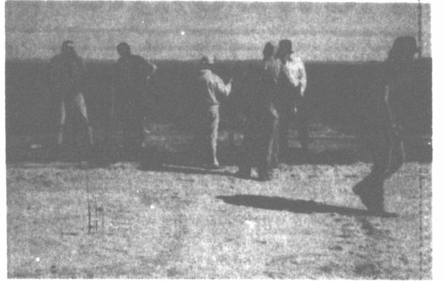
Volunteers begin early work on setting posts for the fence around the cemetery.
