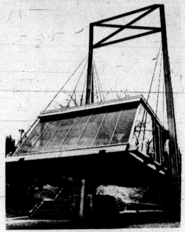
IF YOU LIKE A SUSPENSE HANGUP, this home at the International Exhibition of Domestic Arts in Turin, Italy, is just the thing. It's called the "Tree House," and is of prefab steel, easily disassembled. Vertical beams support the glass-enclosed structure, which hangs from cables. Architect Lorenzo Papi of Florence is responsible.
