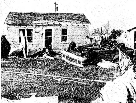
OVERTURNED — A car belonging to Eframes Lopez lays on its roof in the 700 Block of S. Popham in White Deer after a tornado struck the town late Monday afternoon. A car Lopez had in the garage was undamaged.
