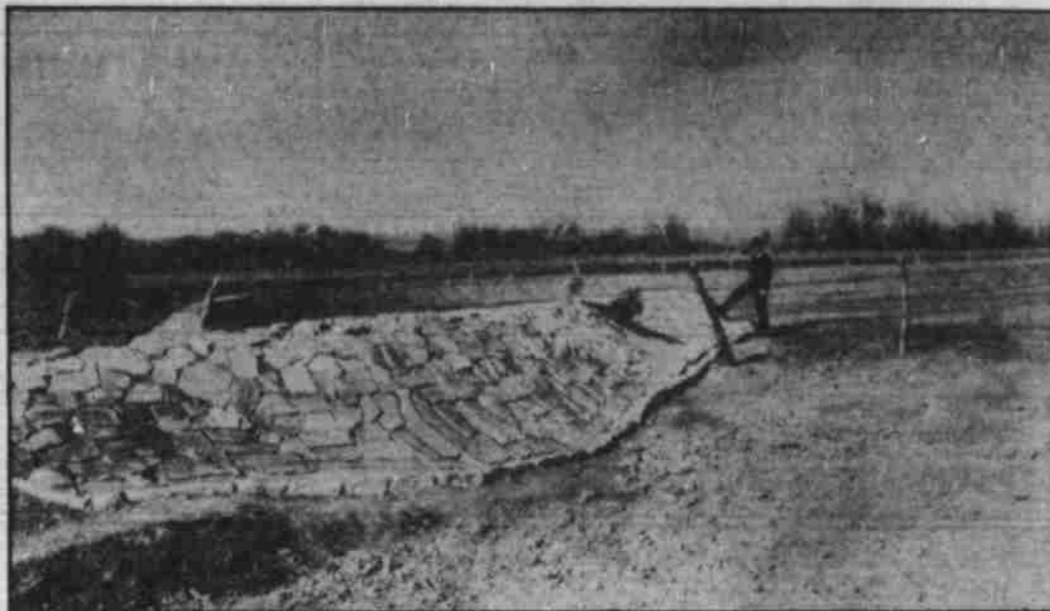
"Dust engineers" have entered the battle to conserve water and top soil in the "dust bowl" by building dikes such as this one being constructed on a farm near Springfield, Colo. Water settles against the dikes, silt settles in the water and the water passes on to be used in irrigation. Dust storms over this area Sunday night and Monday indicated that many such dikes are needed. (Associated Press Photo.)
