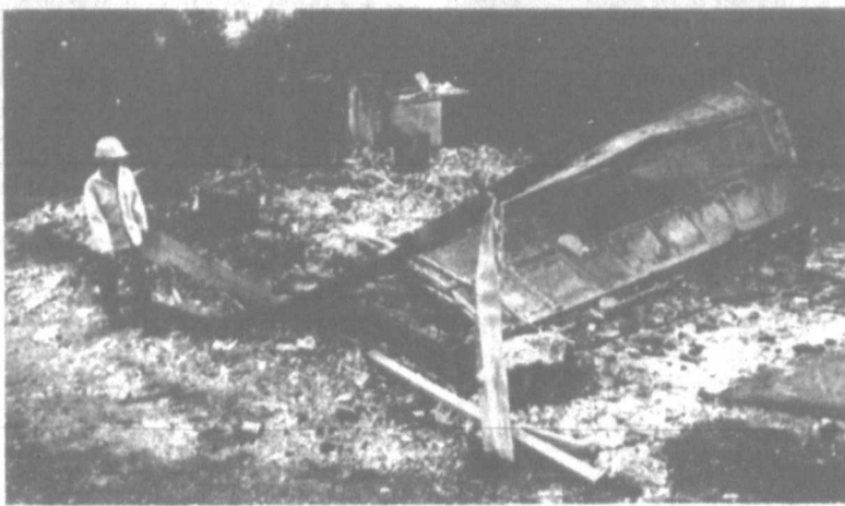
Debris and ashes — all that remain of a house in Lake Wildwood.
