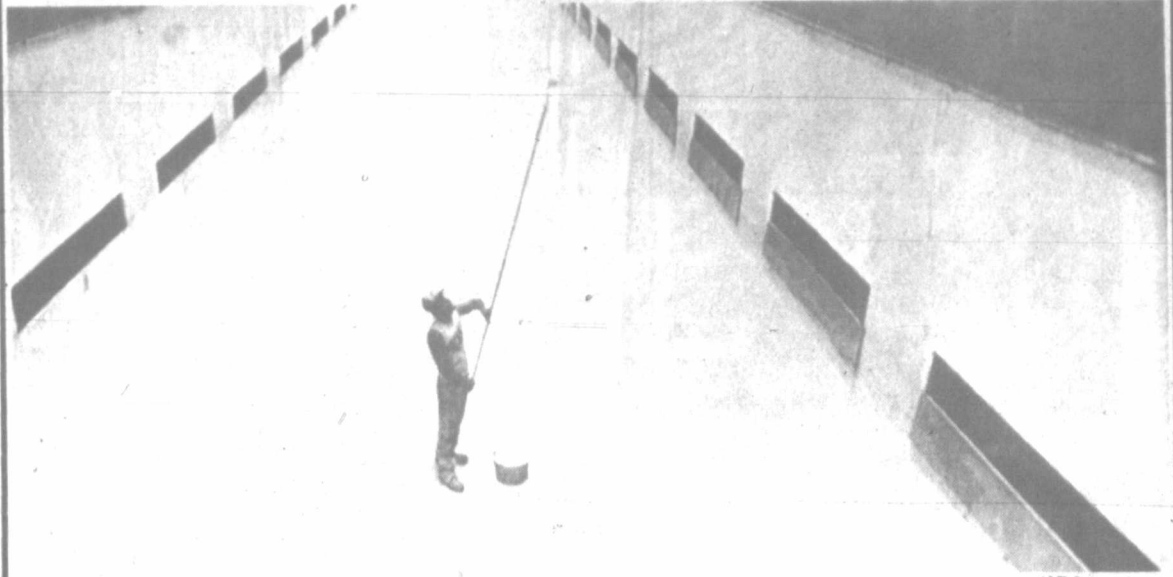
Tim Jones applies white paint to one of 18 long-parts processing tanks at Lockheed Aeronautical Systems Co. in Marietta, Ga.
