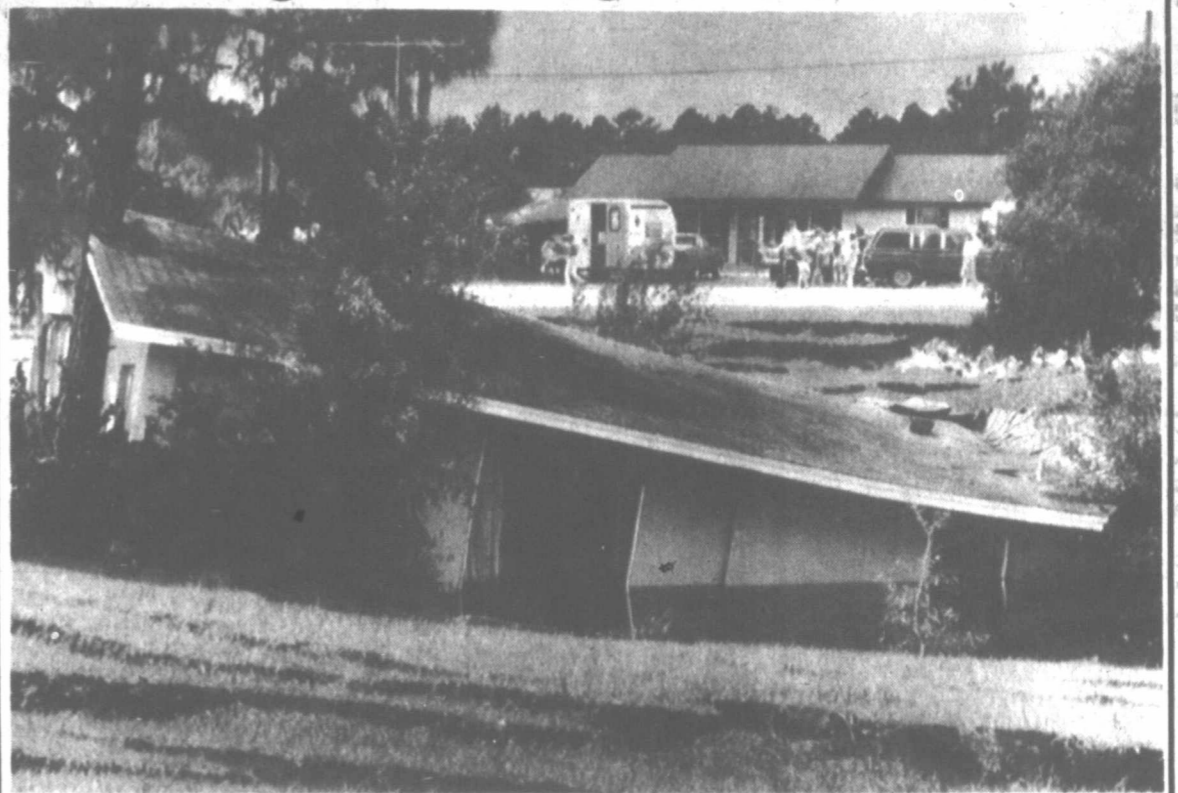
Bill Pivnick's $70,000 home settles further into a sinkhole in Sebring, Fla., Sunday as neighbors gather on the far edge to have a look. Through the weekend the water table began to transform the 20-foot deep acre-sized depression into a pond and neighbors started to talk about moving.
