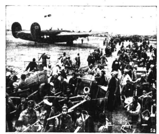
AIRFIELD UNDER CONSTRUCTION—Chinese laborers use buckets, baskets, bar-rows, and carts to carry rock from pile at left to construct an airfield runway bed in China.
