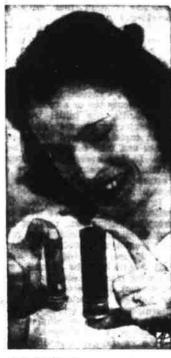
STARTER — Molly Keane compares an airplane starter shell (right), made at Winchester Repeating Arms Co. plant at New Haven, Conn., with an ordinary 12-gauge shotshell. Cartilized furnishes single powerful impulse starting airplane motor.
