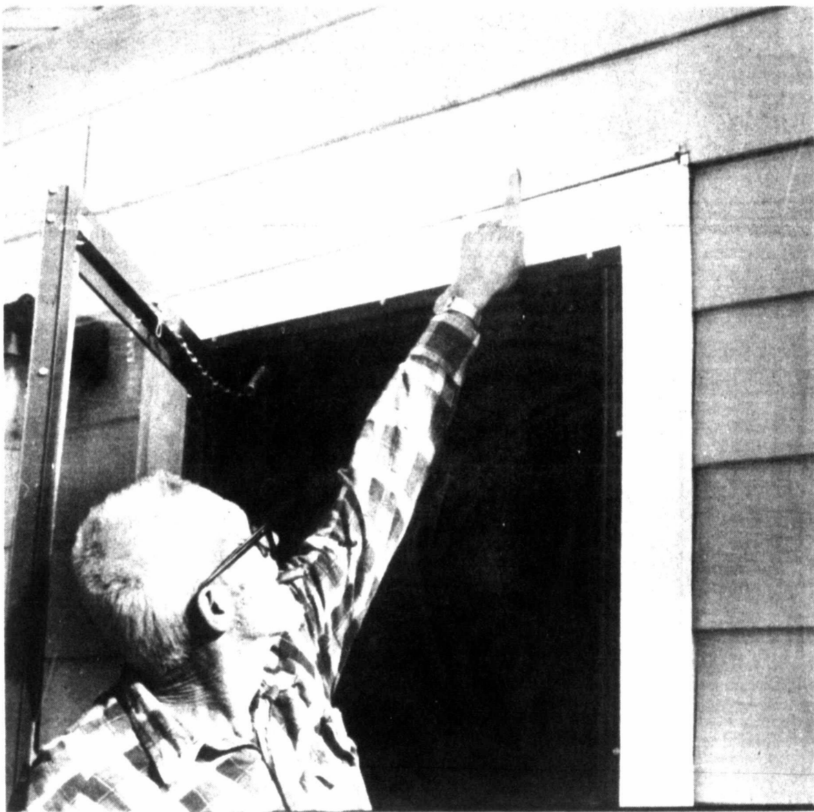
Minton shows damage to outside of Kingsmill home from Celanese explosion.
