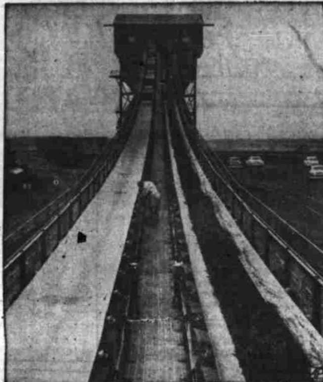
FOR LOADING SPEED — Pennsylvania Railroad's Goodrich conveyor in Philadelphia will carry 3,600 tons of iron ore an hour to freight cars from ships a quarter-mile away.
