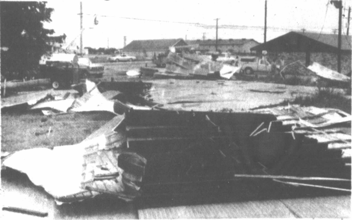
Utility company employees repair downed power lines in the background as wreckage lies in the foreground following a mid-afternoon tornado in Early, near Brownwood, Tuesday. The twister caused heavy
